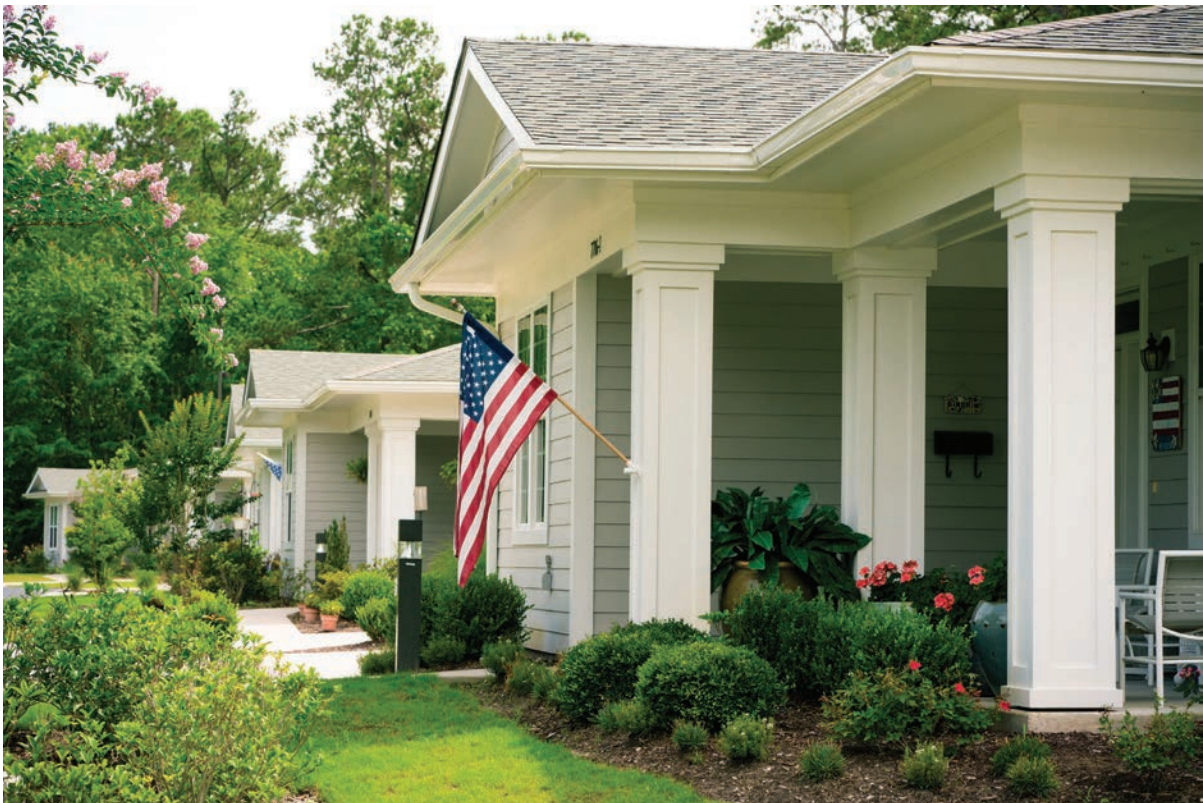
Existing Duplexes Exterior
